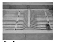
Step 2 Press the heating mat to the insulation and start shooting the plastic tags.
