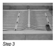
Squeeze out the glue with the piece of duct tape toward the insulation at the mat level and wait a few seconds.
