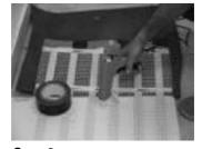
Step 2 Press the heating mat to the surface and apply a small amount of glue.
